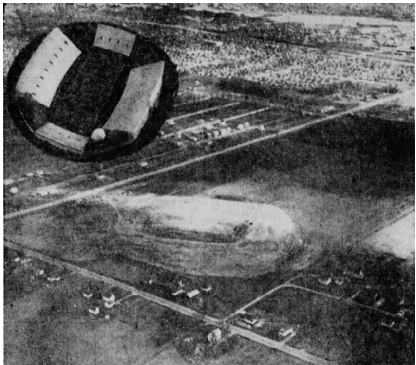
Work Continues on Packers' New Home —Here is an aerial view of a bulldozer at work on the site of the Green Bay Packers' new 32,000-seat stadium at the corner of Highland Ave., and Ridge Road, with a model of how it will look in the inset in the upper lefthand corner. The Packers are scheduled to play their league games in the new stadium next year.
